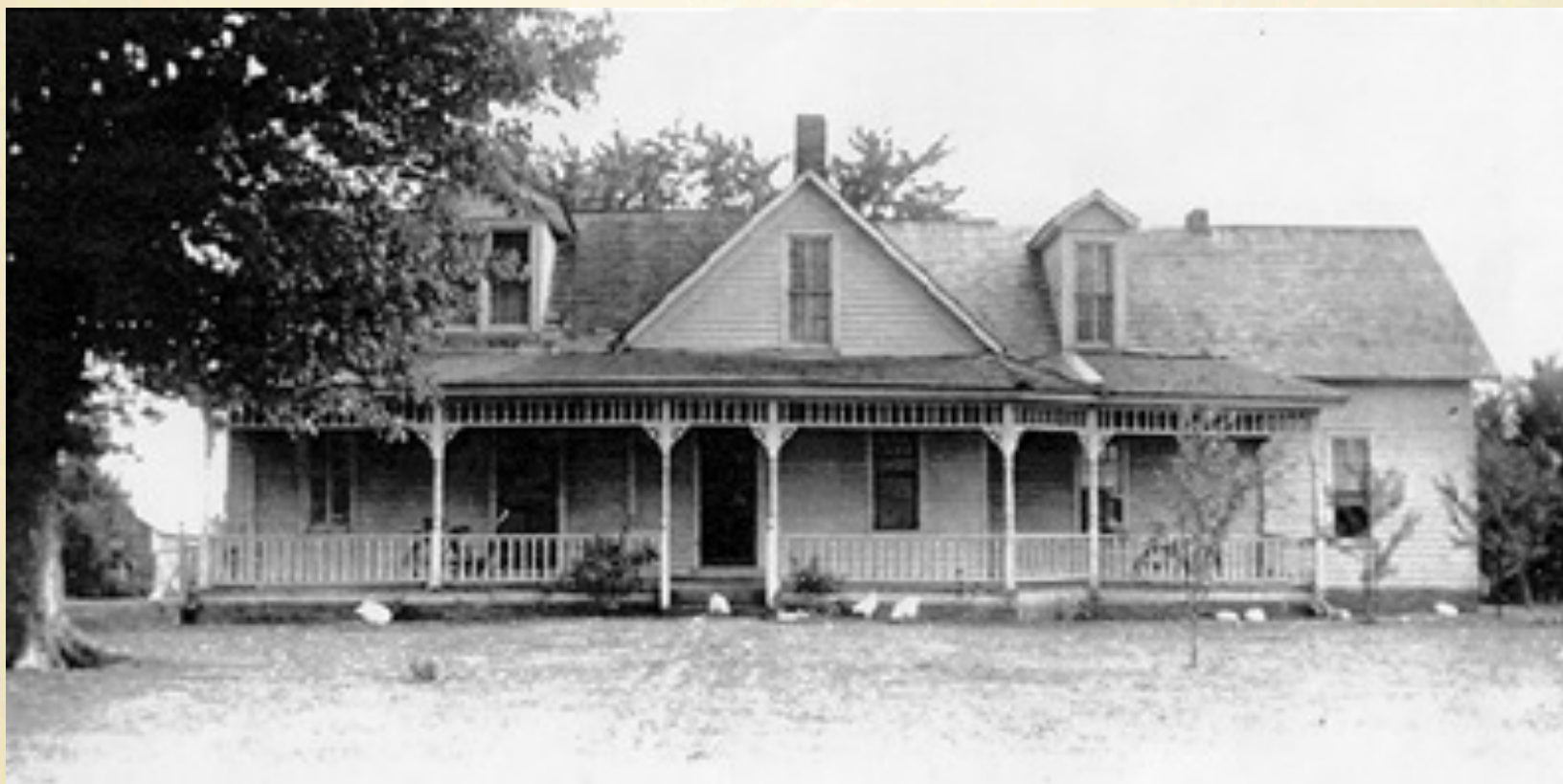
O'DAFFER FAMILY HOUSE NEAR WELDON, ILLINOIS
