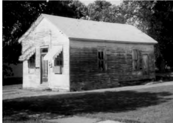
Old Weldon Public Library, now abandoned
